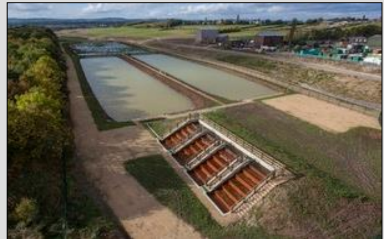
British Coal Authority: Wasserbehandlung Derbyshire
